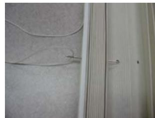
Fig. 3 Starting at top rail, thread string through holes as illustrated on diagram
